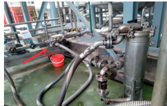
Liquid Trap in a flow line
